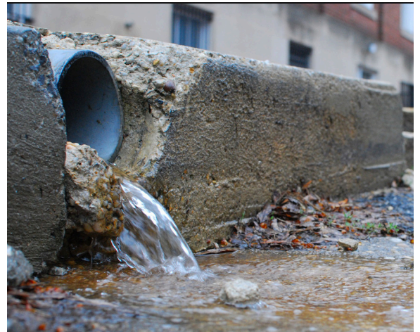
Stormwater outfall
